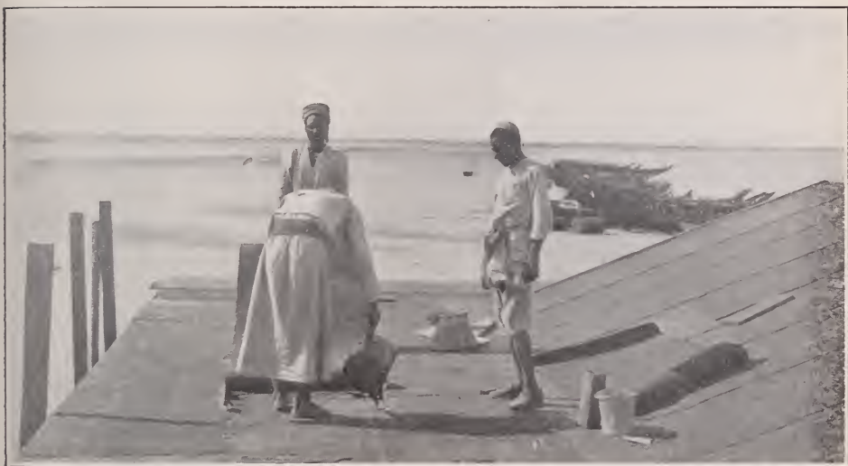
ROOFING THE HOSPITAL.
